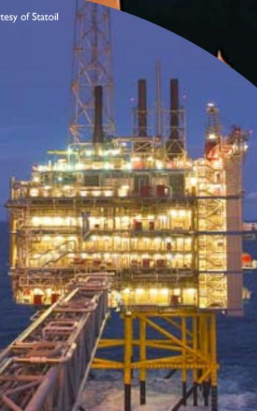
Carbon capture and storage is feasible. Carbon dioxide extracted from gas production on Statoil's Sleipner West field in the Norwegian North Sea is stored 1,000 metres below ground instead of being released to the air. The process, in use since 1996, sequesters about 2,800 tonnes of CO<sub>2</sub> every day.
