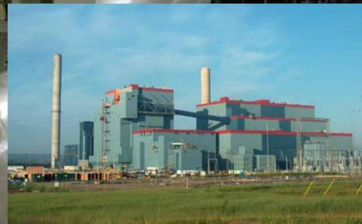
Genesee 3 (G3), the third unit at the Genesee Generating Station in Alberta, is the first facility of its kind anywhere in Canada. Equipped with \$90 million in clean air technologies, G3 features the first-time use of a supercritical boiler to produce electricity more efficiently than traditional coal-fired generation.
